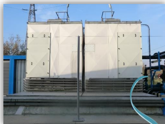
Installation of large polyester doors Increased accessibility
