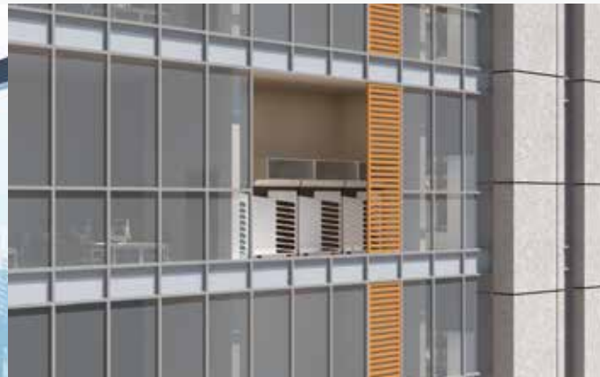
The outdoor unit is hidden inside the building without affecting the overall image of the building
